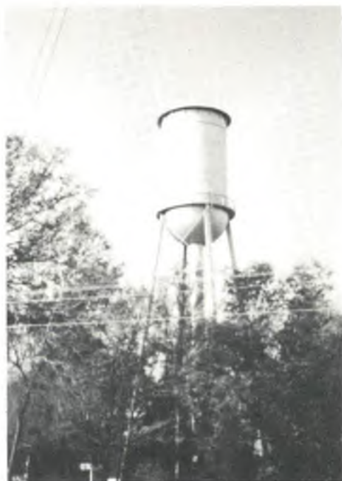
The first water tower built in Brookings. Located on 4th Street, it is still in use.
