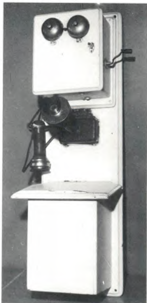
Many early telephones were made by the Stromberg-Carlson Company. A few of the instruments were still in use when the telephone department converted to dial telephone in the 1950s. This telephone was approximately 65 years old when it was photographed in 1958. It was still in working order and was used by Mr. and Mrs. Ed L. Merchant of Brookings until 1956.
