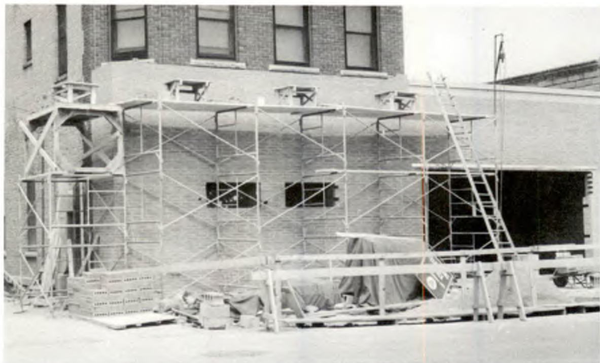
Telephone building under renovation in 1957.
