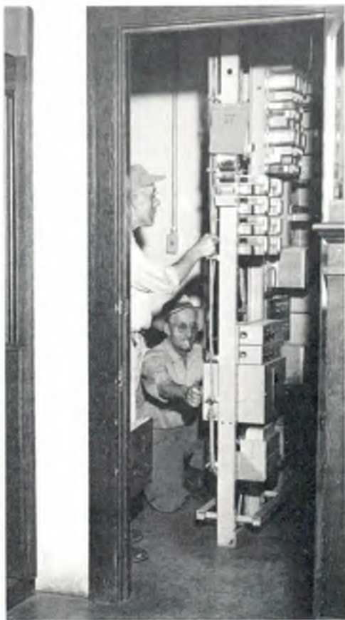
Morse Johnson, Watertown, and Chet Robinson, Volga, working on toll terminating equipment.
