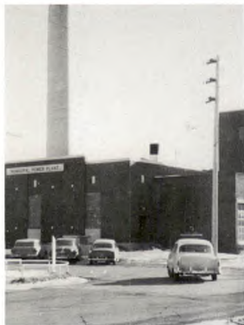
The power plant as it appeared in the 1950s and until it was razed in 1980.
