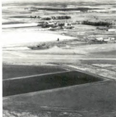
Stabilization ponds in the late 1960s. Old sewage treatment plant to right of ponds. Lagoons in dark sections.
