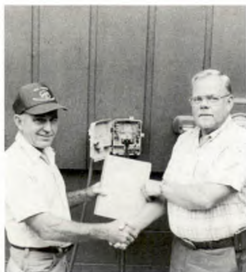
From 1989-90 a Network Interface Device was installed at every home having telephone service. Customers could determine if a problem was in their equipment or with the telephone cable. Shown here are installer Bob Tusher and outside plant supervisor James Lee.
