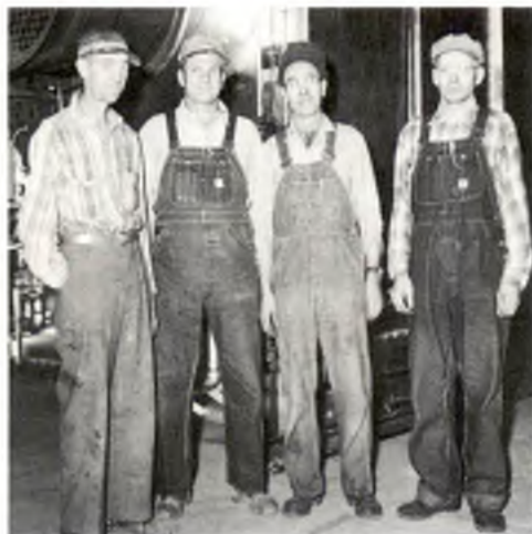
Power plant crew in 1950s. From left, Marvin Jensen, Jack Horner, Walter Johnson, John Pickering.
