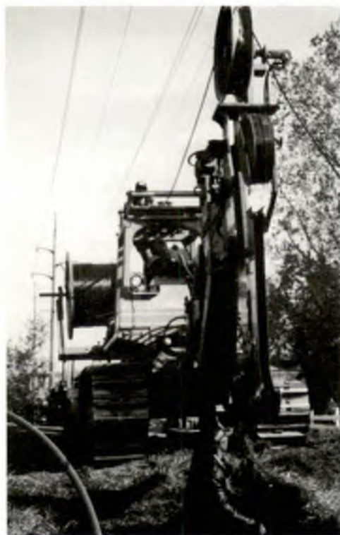
Installing fiber optic lines near Sioux Falls in 1989.
