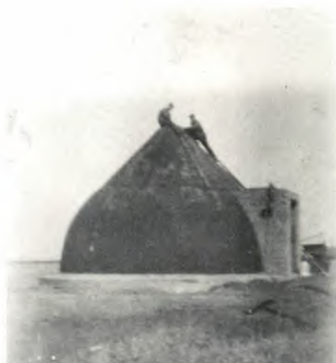
A community supply of water was one of the concerns of people who settled in Brookings. From the first water was plentiful, but making it accessible was a problem. Pictured here is the old well house.
